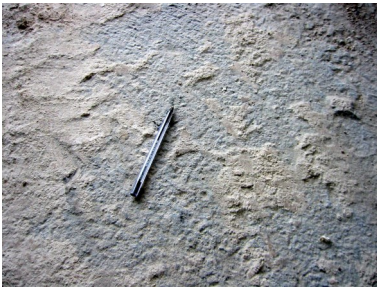
Magnesite residues on a floor
